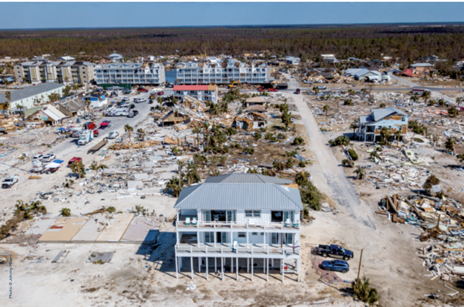
➔ House still standing after Hurricane Michael 2018, Mexico Beach, Florida
